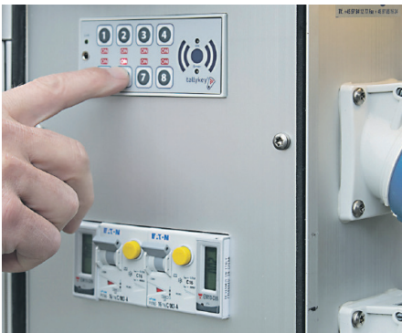
Power self-service with individual code. Pay according to consumption or in packages. No consumption without payment.
